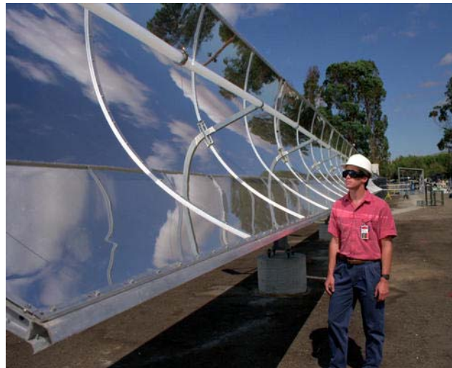
Figure 8: Previously used solar trough, used for producing electricity. Image found at: http://thefraserdomain.typepad.com/photos/uncategorized/2007/07/28/solar_trough_3.jpg
